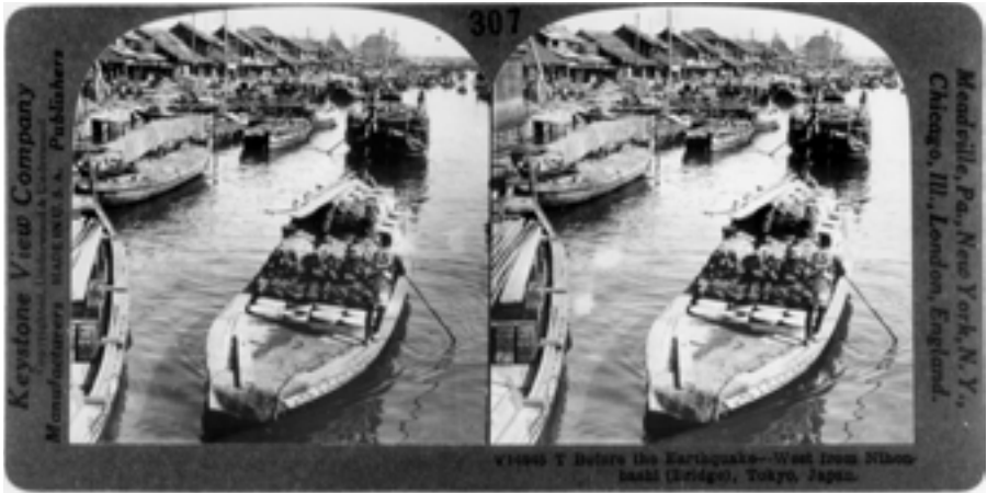
Figure 28. “Before the Earthquake—West from Nihonbashi (Bridge), Tokyo, Japan.” American stereopticon slide, ca. 1925 (Keystone View Company, no. V14945). Reproduced with permission of the Morita Photo Laboratory.
